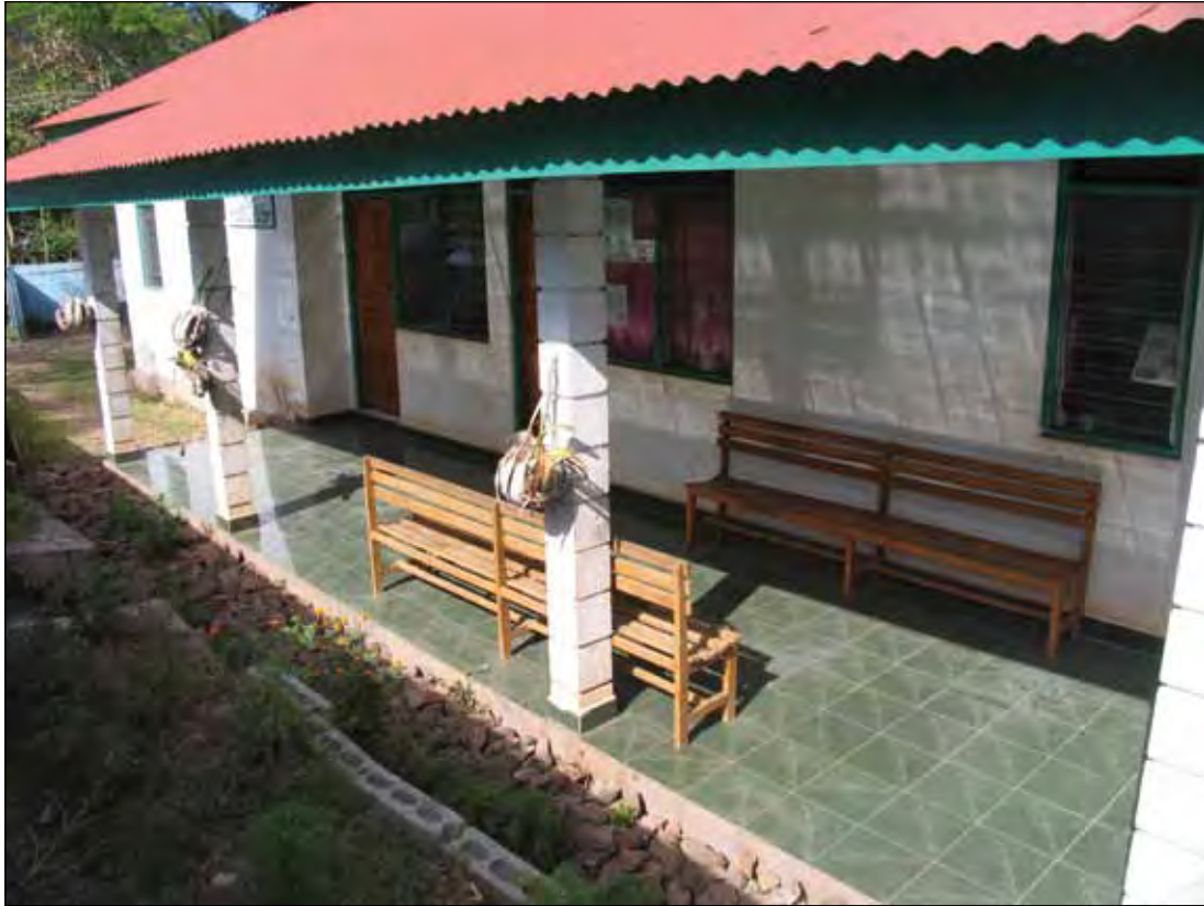
The government run health clinic is the largest building in the area, Sarelari, Luro, October 2007
